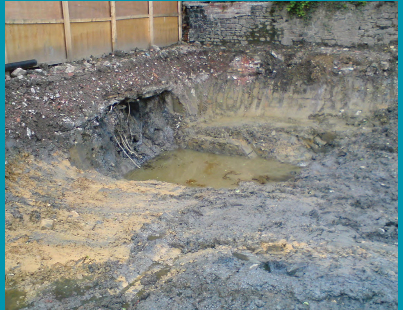
An excavation shows soil contamination at an industrial site in England. In the early 2000s, researchers developed a method to smolder hazardous organic liquids such as oils, solvents, and coal tars that were found in the soil.
