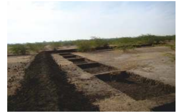
Chouka system (set of small-scale interlinked percolation ponds)
