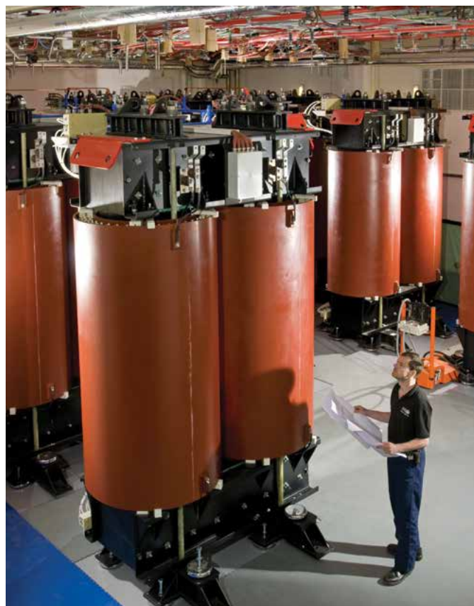
Steve West inspecting the new ISIS MMPS main chokes during installation in R6A back in May 2009.
