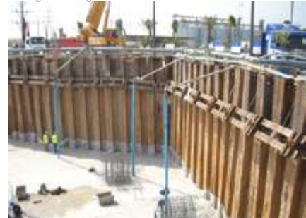
Waling beam with ground anchors
