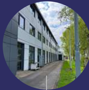
Block A - re-clad
