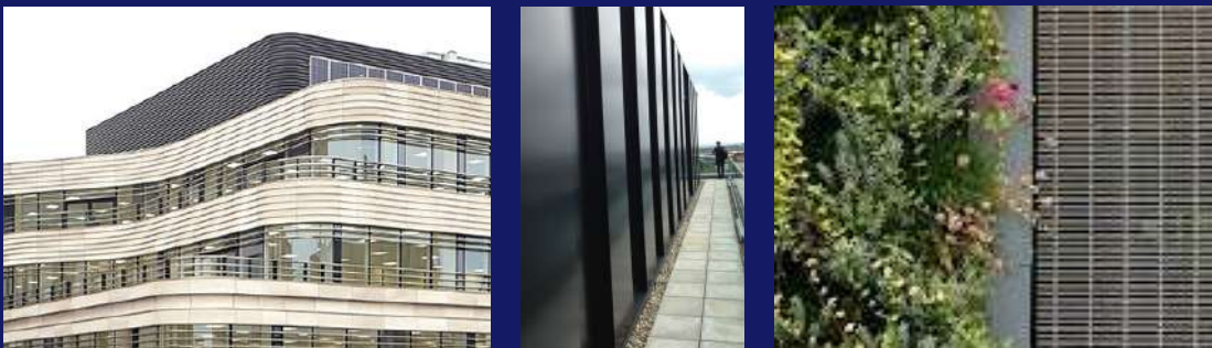
Precedent examples of screening of roof plant
