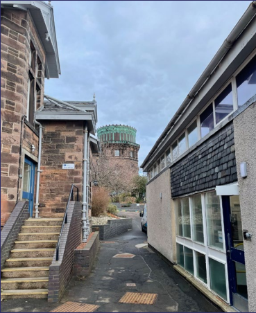
Villas and workshop
