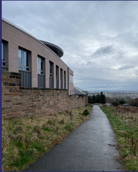
Reconstructed southern wall
