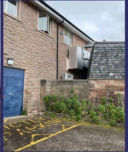
Service entrance to workshop
