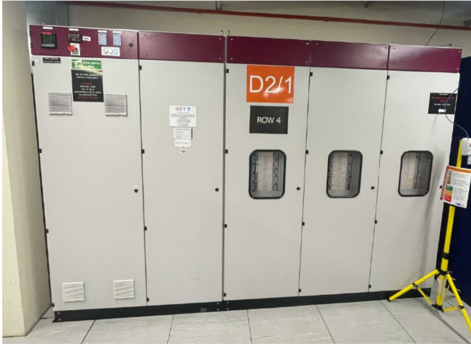
Figure 6: Existing PDU example
