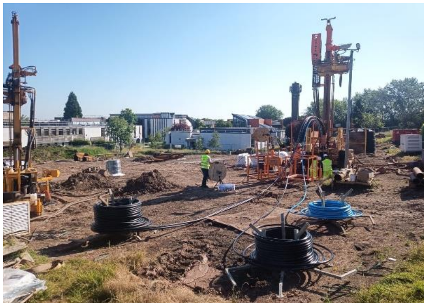
Image: Installation of heat pumps at BGS Keyworth. Credit: BGS
