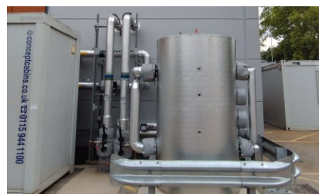
Geothermal heat pump at BGS Keyworth Credit: BGS
